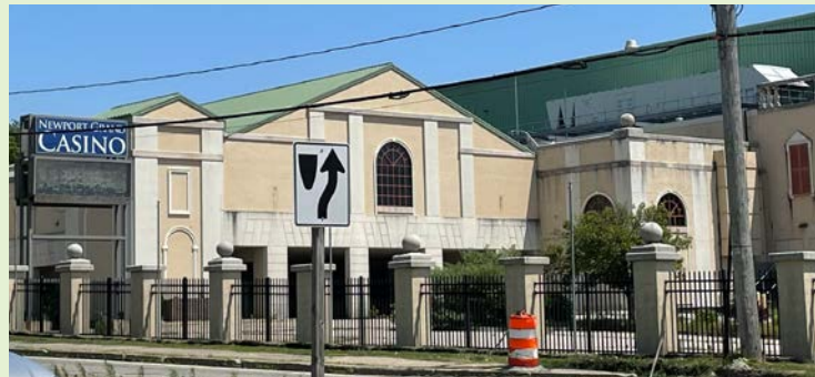
Shuttered former casino property at the center of the Innovation Hub Photo by Rex LeBeau
